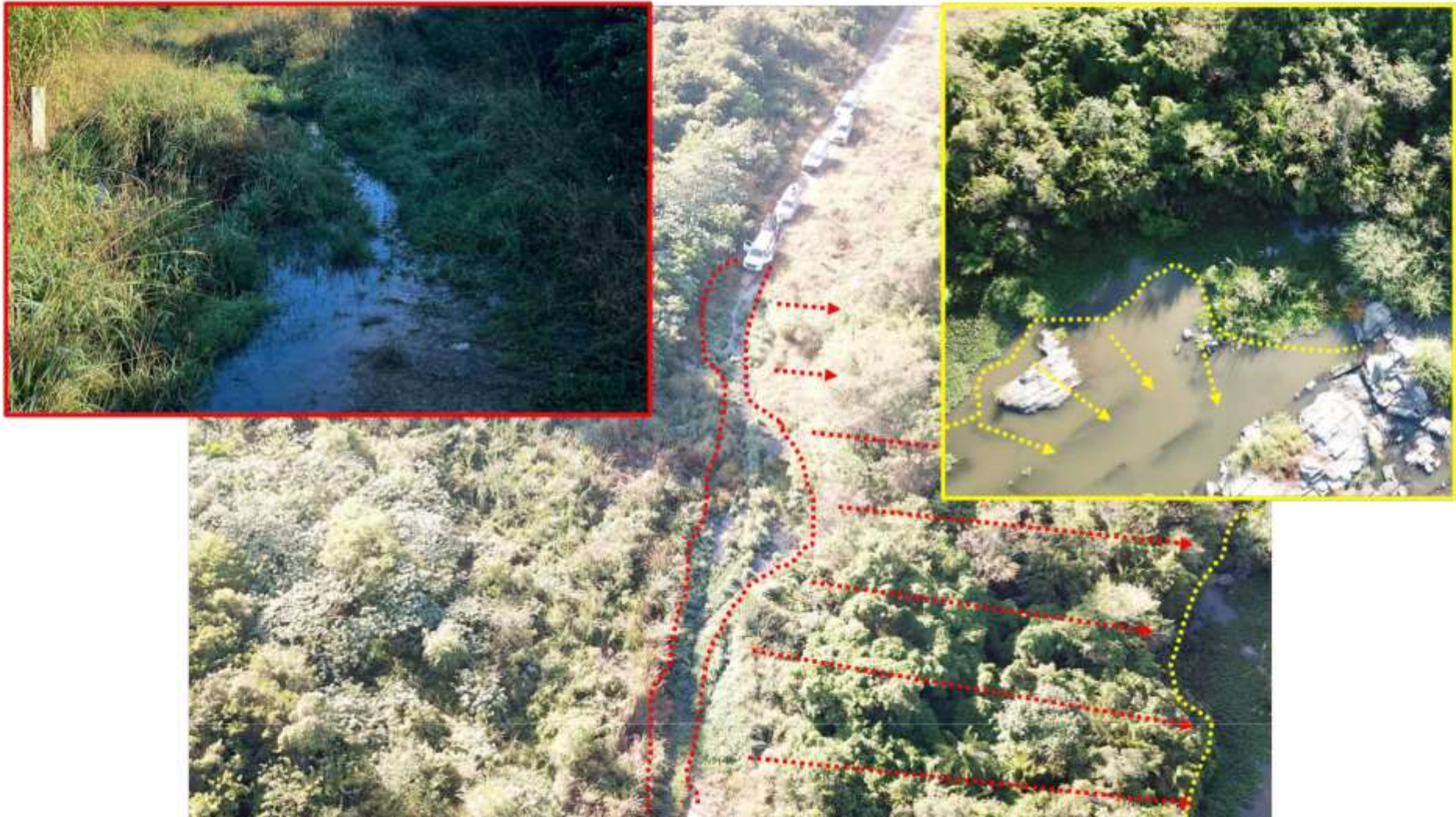
Figure 1: Accumulation of raw sewage along the access road to the Lower Buffalo Reach and the concentrated hyacinth along the margins
